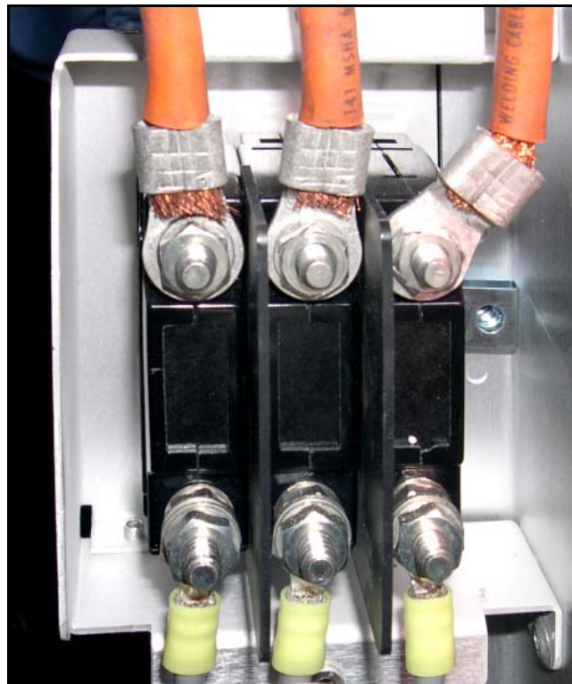
Figure 2-3 3 Phase Connections to CB1
