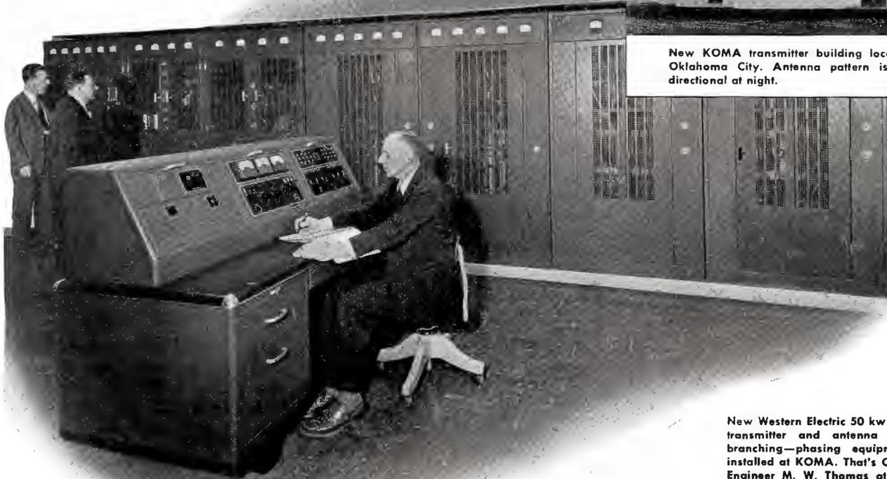
New Western Electric 50 kw AM transmitter and antenna line branching—phasing equipment installed at KOMA. That's Chief Engineer M. W. Thomas at the control desk.
